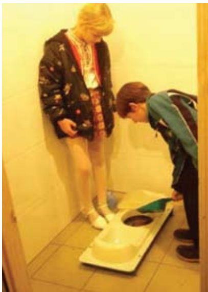
A trowelful of a mixture of ash, sawdust and sand is put in after every use, to enhance drying and help early destruction of pathogens
