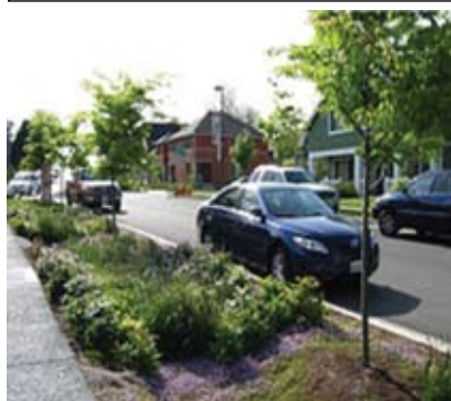
Swales are roadside depressions – designed to reduce storm water runoff and encourage local water table recharge
