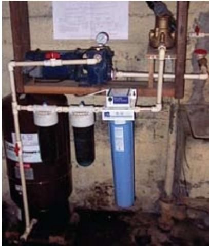
Purifying Rain water - Two particulate filters in series, rated at 20 and 5 micron particle size & an ultraviolet light sterilizer.
