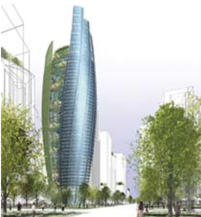
"The tower of tomorrow" is full of biomimetic functions including: self-cleaning interior spaces (plants filtering the air), the aerodynamic shape diffusing wind load on the facades, and a water reclamation system redistributing greywater for toilets and other non-potable systems.
