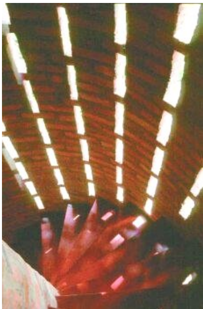
A stairwell in a residence in trivandrum has a perforated brick wall creating
