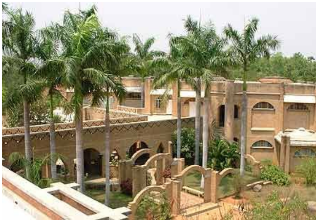
The award winning visitor's Centre at Auroville made with compressed earth blocks is one of the most attractive and comfortable buildings in south India.
