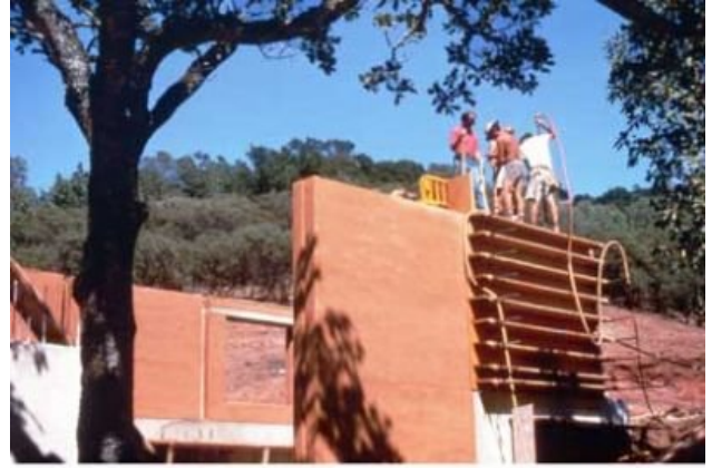
USA, California - Project by Rammed Earth Works
